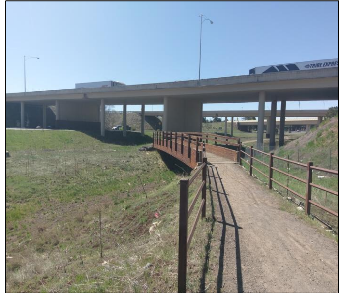
Figure 1: Existing Structure Facing South
