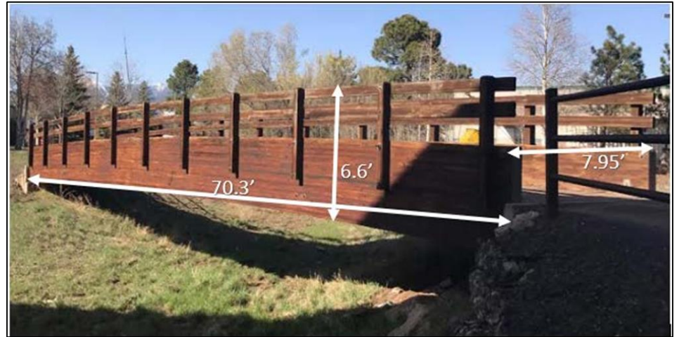
Figure 3: Dimensions of Existing Structure
